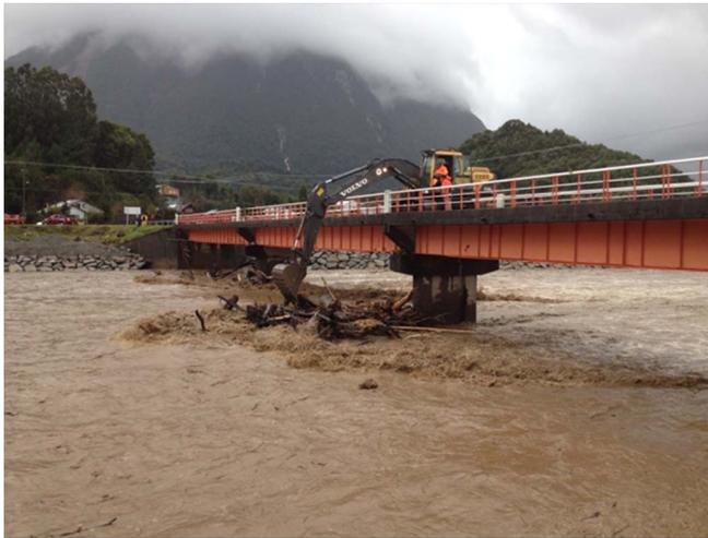
Fig. 14. photograph showing removal of clogged LW at the bridge of Chaitén village during a winter flood in 2015 (photo provided by El Llanquihue newspaper, daily paper of Puerto Montt city).
